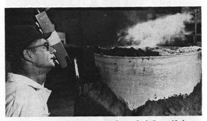
STILL-HOT CASTING emerges as the sand of the mold drops away. Small rod-like element sticking out of sand at left is one of the "down sprues" through which the molten meal flowed through to the "gate" in the bottom of the mold.
